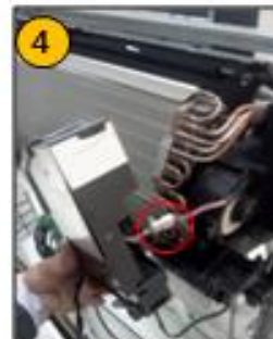
Disconnect motor connector before completely removing it
