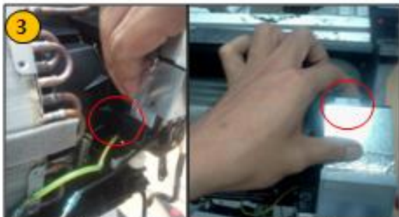
By releasing the 2 hooks (picture) take out the control box.
