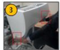
Grab the lower parts & remove Front assy from the unit
