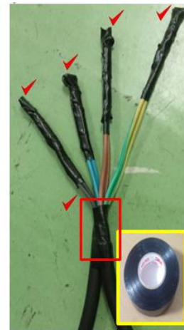
Insulation of each line by tape
