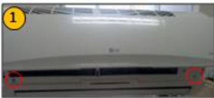
Lift the inlet grille and remove 2 screws.
