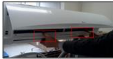
Hold the parts (picture) and slightly lift it up until it is removed from its hook. ("Ttuk" sound)
