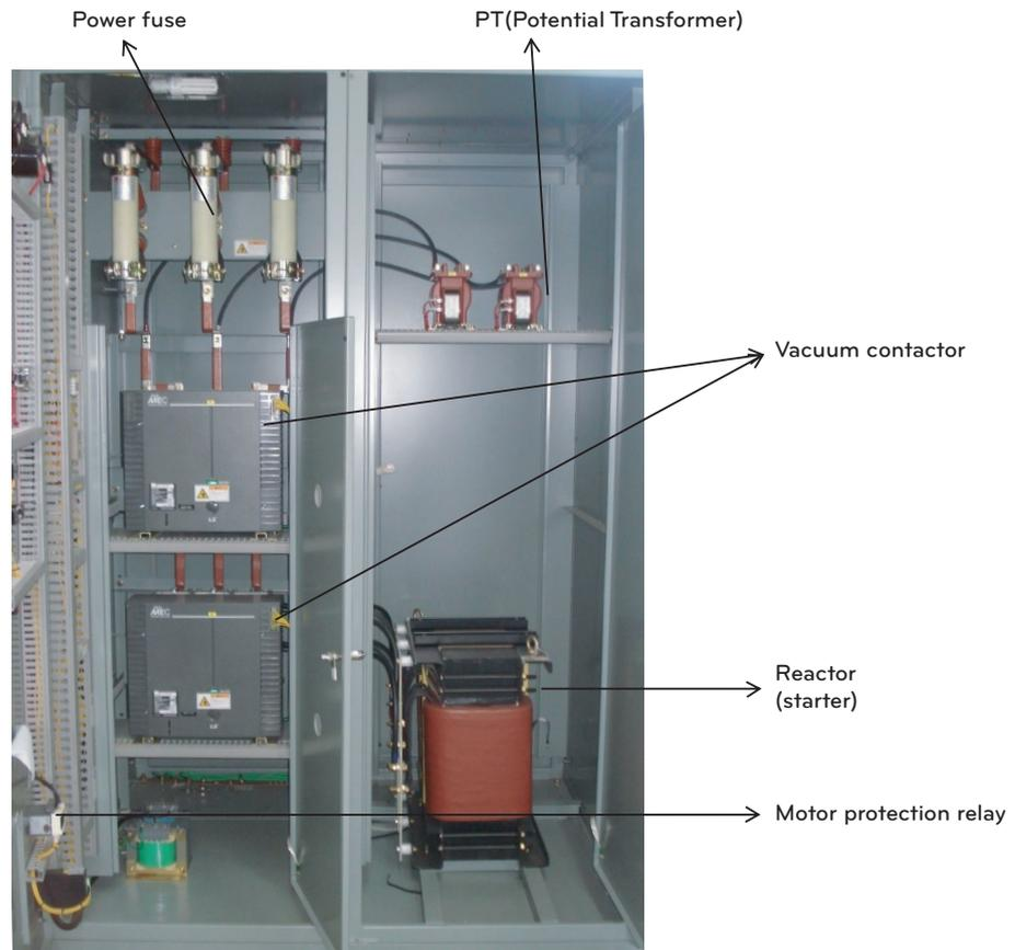
Figure 15. 6600V Reactor start-up type
